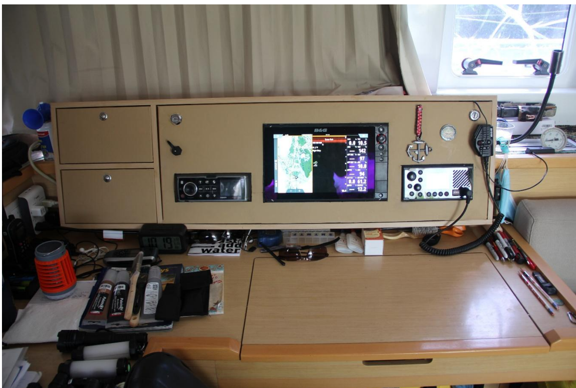
Salon navigation/instrumentation electronics powered up
